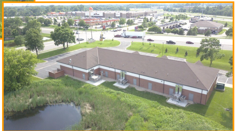
Facing Fleet Farm - Signalized intersection
