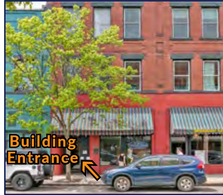
View from across Broadway Street
