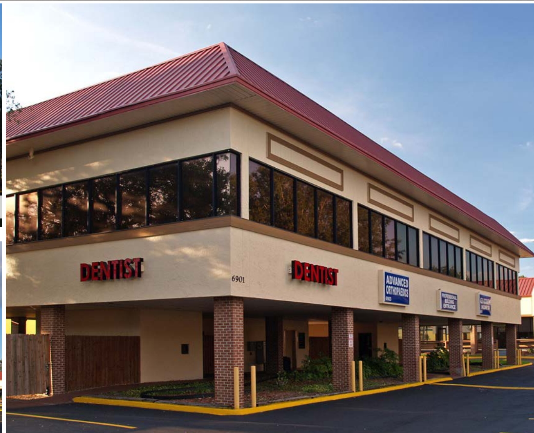
Two story office
