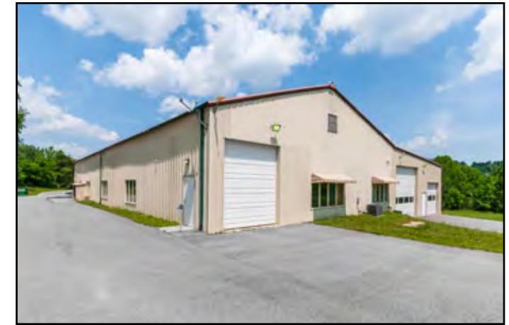
View from southwest corner showing 3 of 6 roll-up doors, and windows at office area
