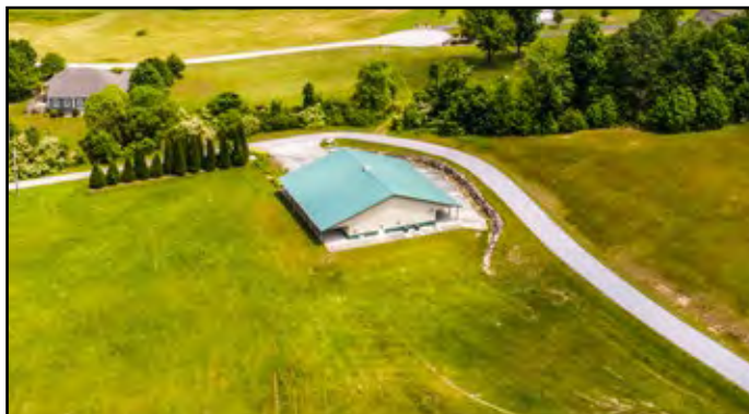
Aerial over the Event Center
