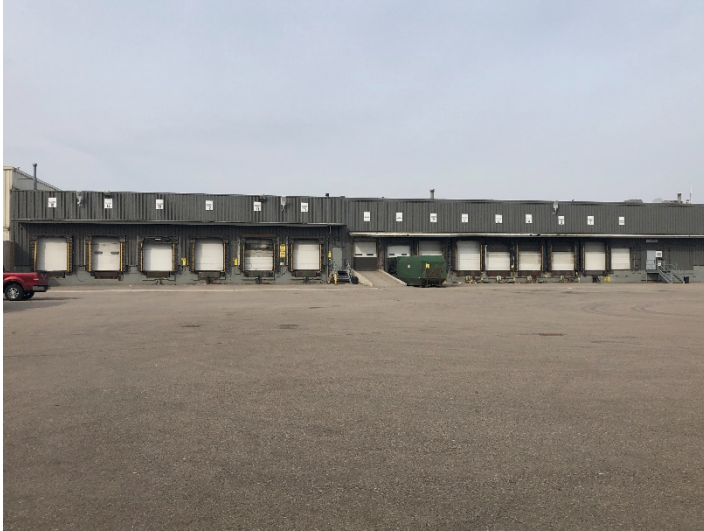
240' deep dedicated truck court/yard
