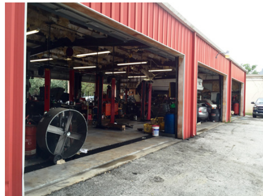
BACK OF BUILDING
