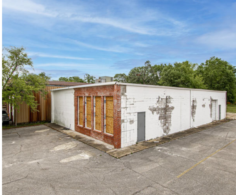
Solid Masonry Construction
