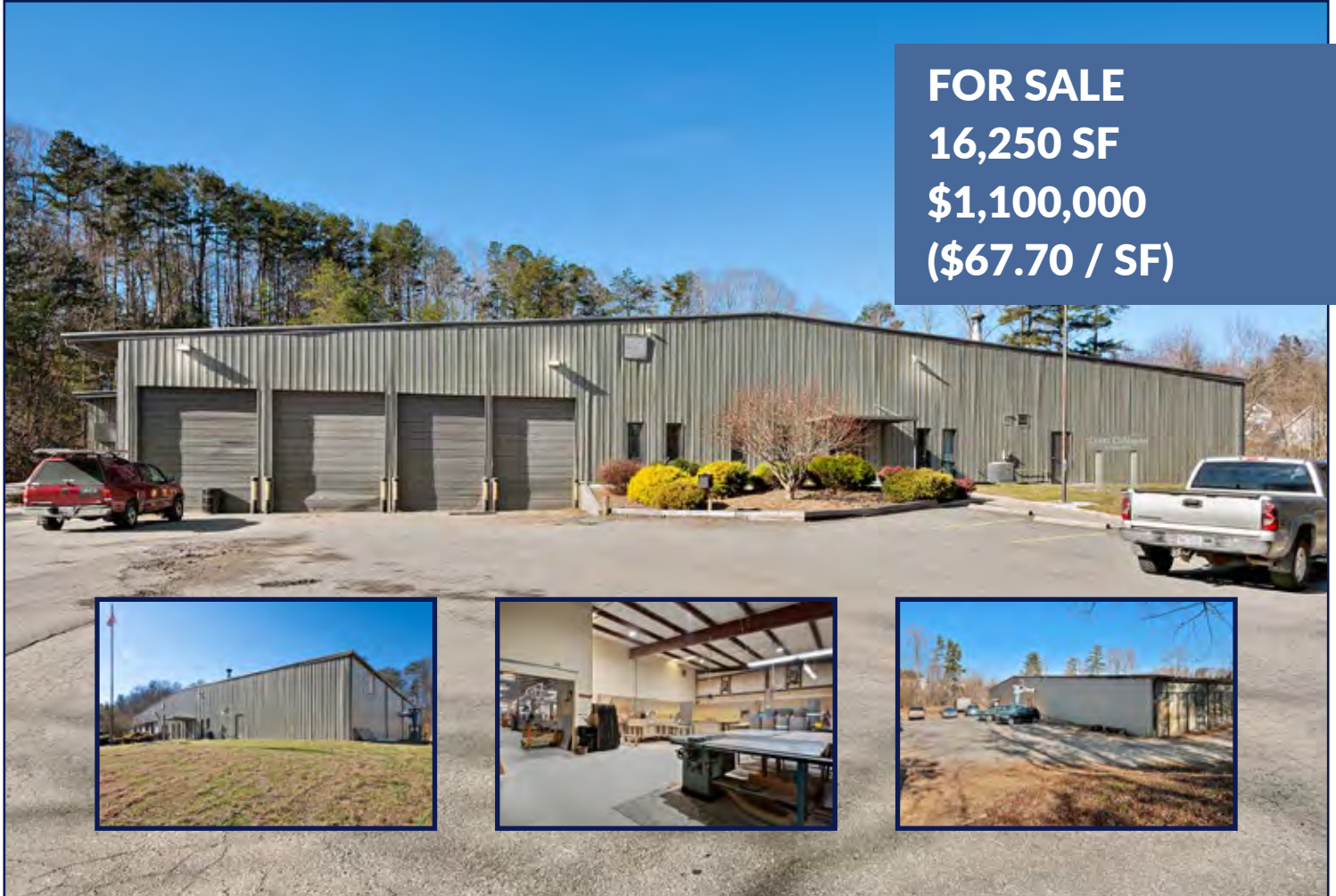
Front of building; Insets, left to right: The facility as seen from the north corner; The processing room; Rear parking area
