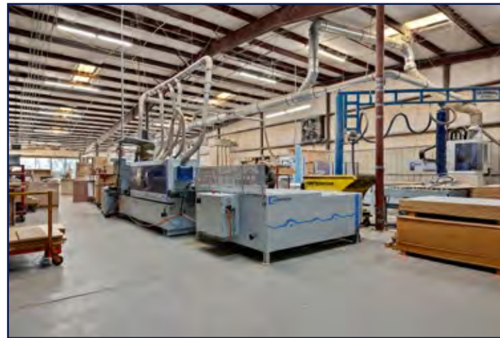
Main manufacturing space
