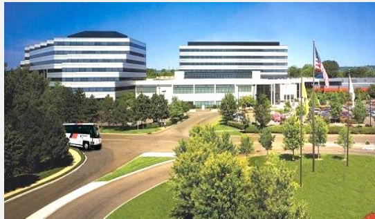
On-site – NJ Transit bus stops
