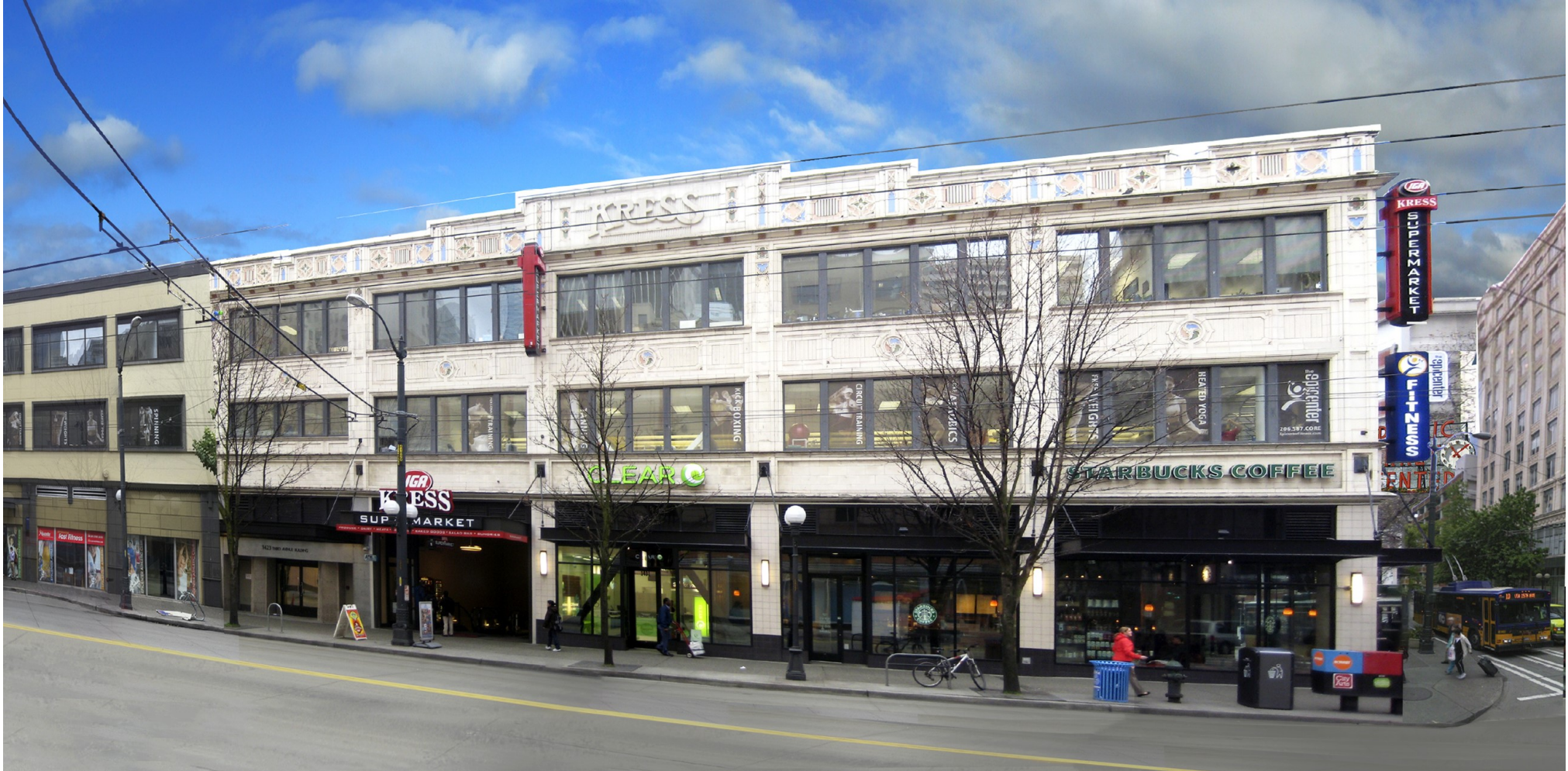
View from Third Ave looking West
