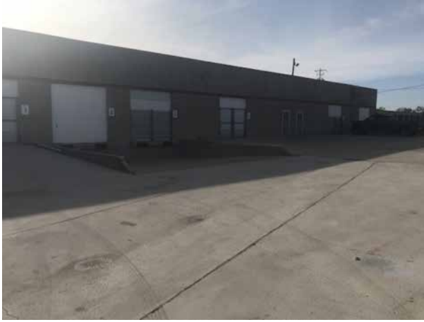
Loading Area with 3 Dock-High Doors
