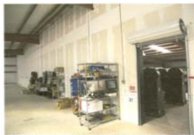
Interior View of the Central Demising Wall Within The Warehouse Area.
