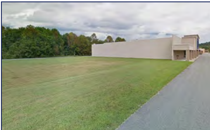
View from end, looking toward Peebles
