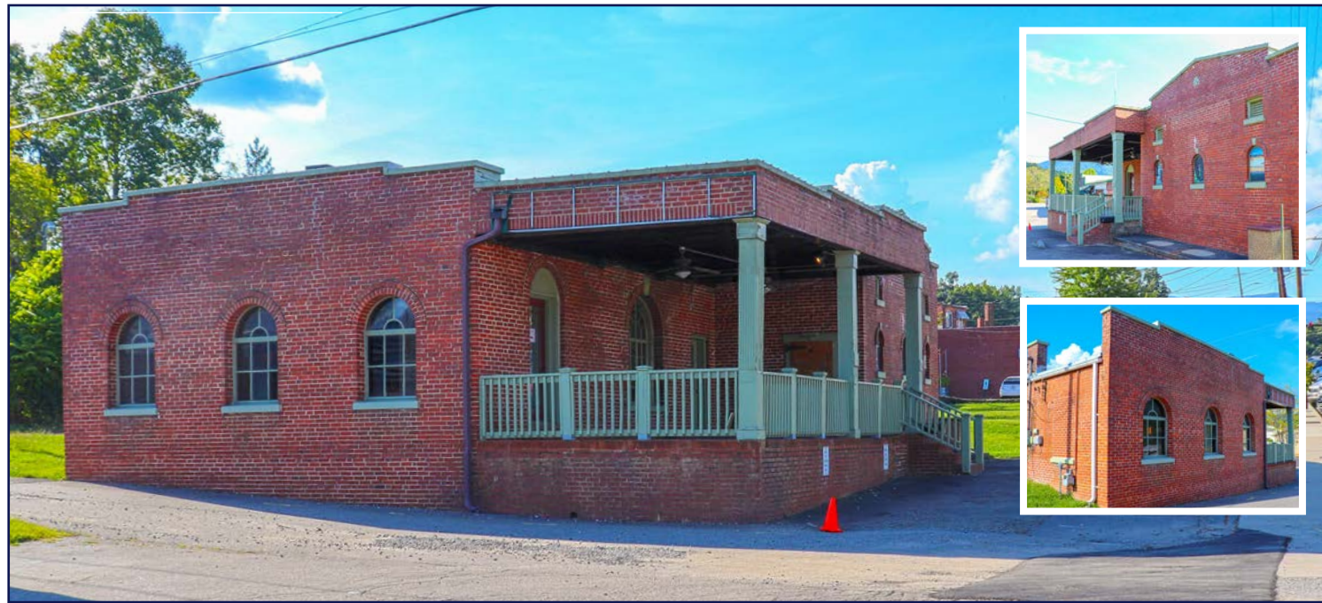
Current view of Icehouse building
