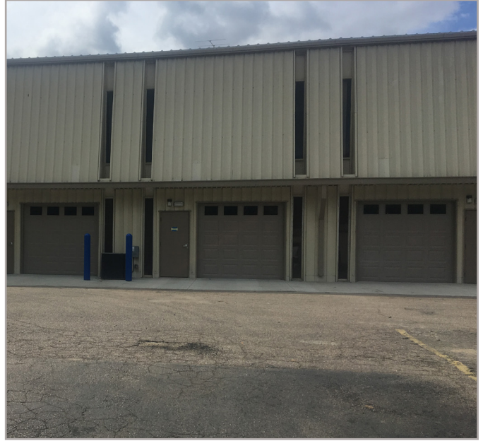
New roll-up doors to fully conditioned warehouse suites
