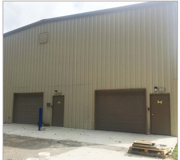
New entry doors with keypad access
