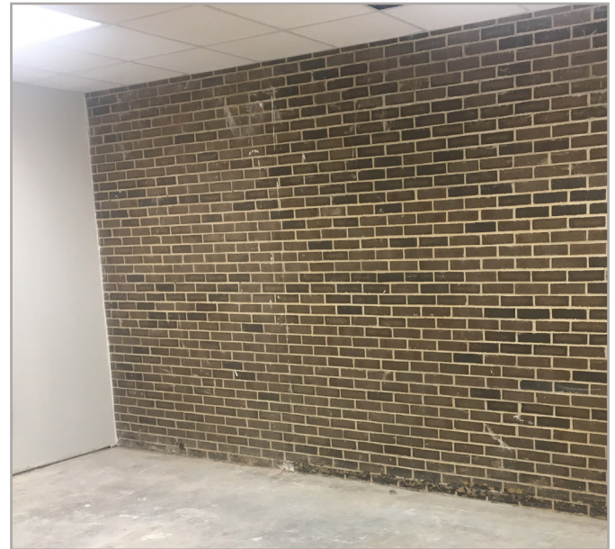
New ceiling grid
