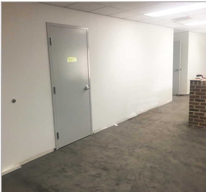
Lobby upgrades including new paint, carpet and ceiling tiles
