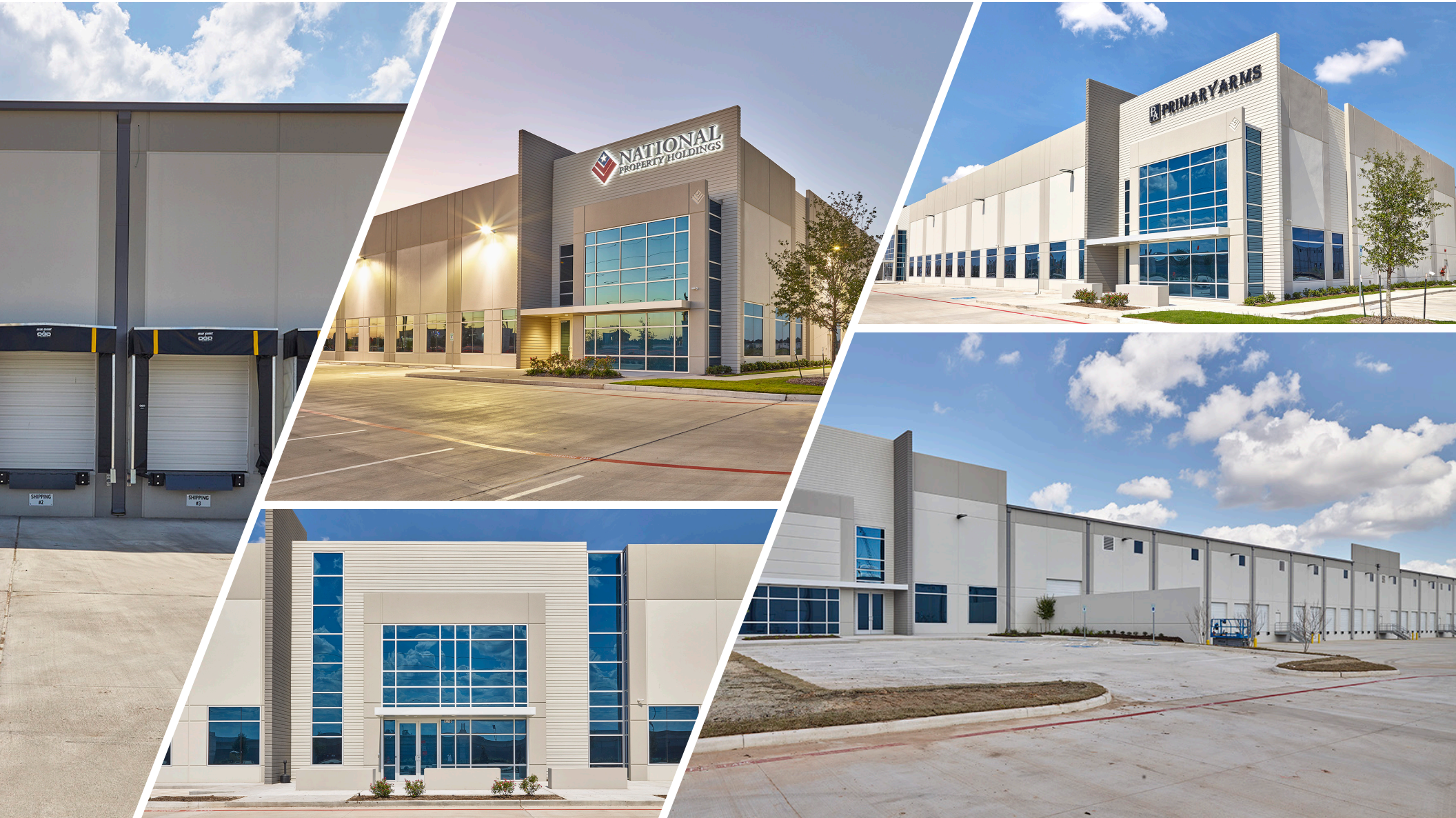
CLOCKWISE FROM TOP LEFT: Dock high loading, LED exterior lighting maintains the business park well lit in the evening, Prominent tenant signage along Beltway 8, Front load space configuration, Substantial office entrance
