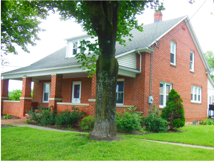
Brick office building currently leased to Blosser Electric
