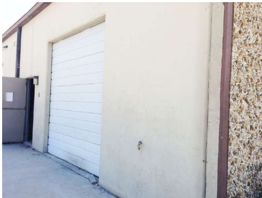
High-pressure water bib
