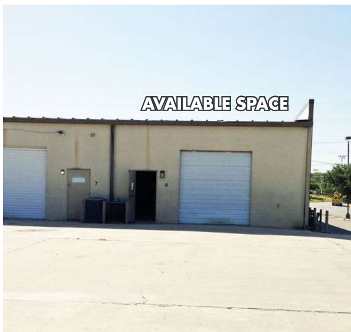
Large parking area located behind warehouse area.
