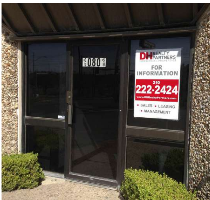
Entrance to 10801 / End-cap Space
