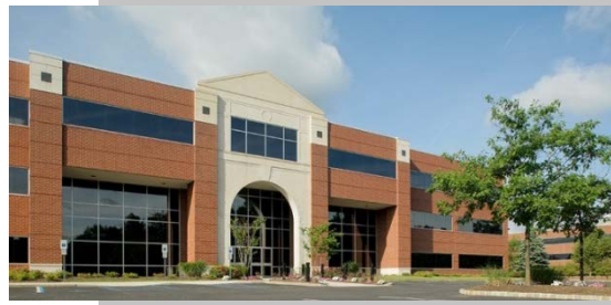
CenterPointe II 1160 Route 22 East, Bridgewater, NJ
