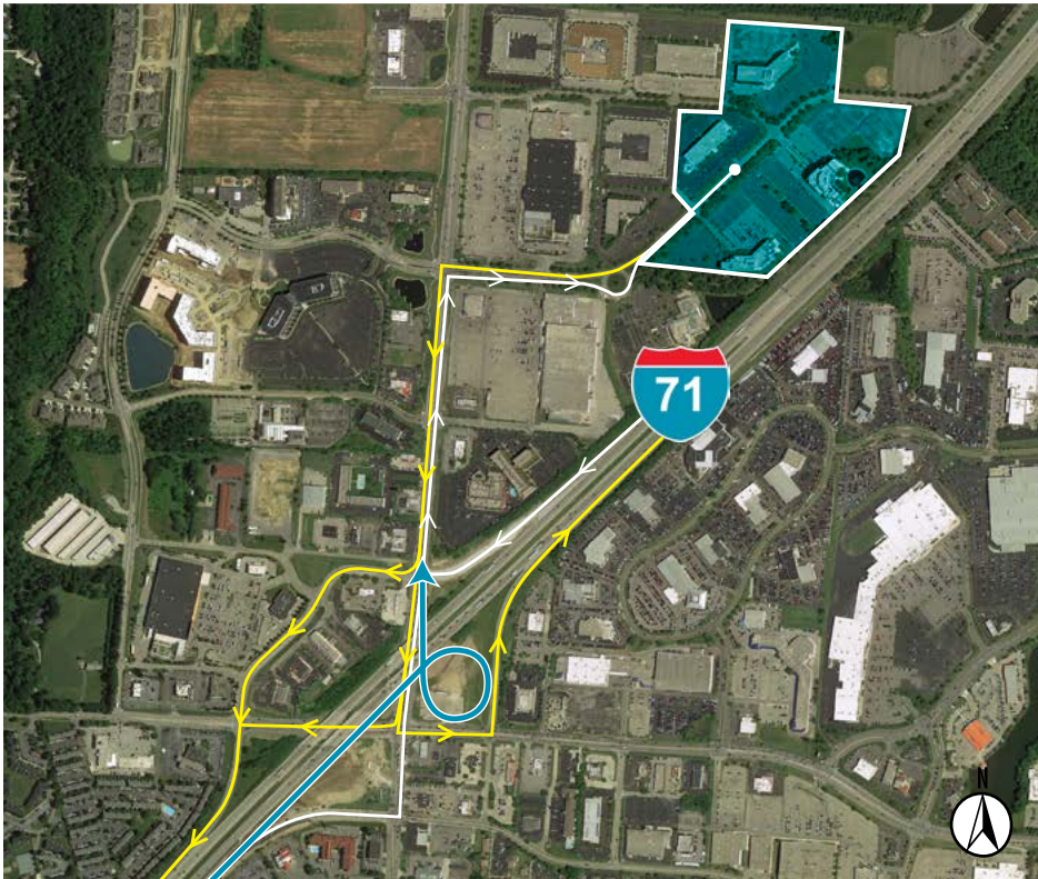
New I-71 Exit Ramp
