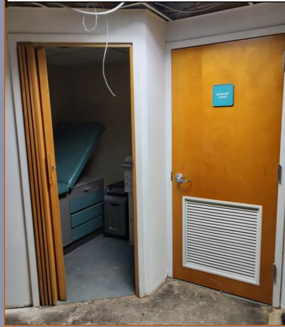
Exam room/closet storage.
