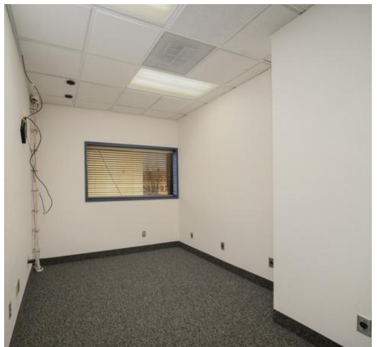
Suite 204 - Server Room
