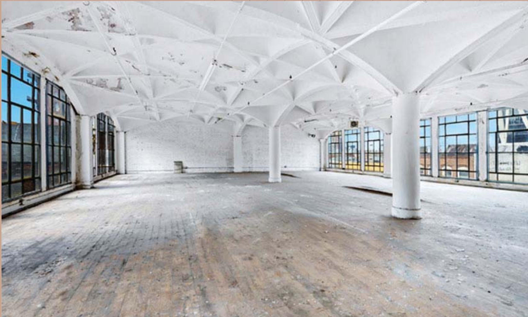
Entire 2nd Floor - Existing Conditions
